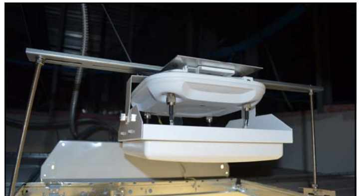
Mount Installed Above Ceiling Tile Grid With Cisco AP 3702e and TerraWave Antenna (M6060060MP1D43602)
