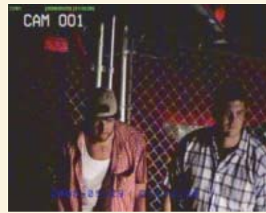
Photo 4. A pan-tilt-zoom camera mounted on a tower leg or on the roof of the shelter with non-penetrating room mounts allows closer observation of intruders.
