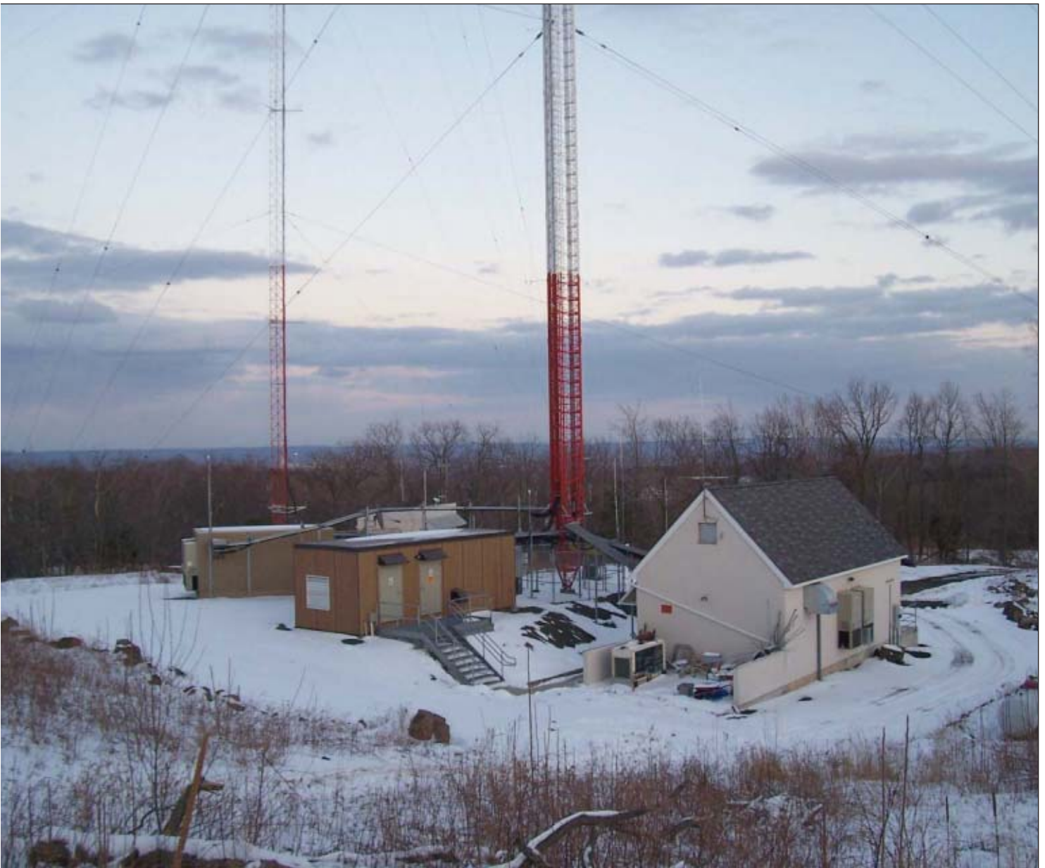
It's quiet at the Marlin Tower antenna site, but on nearby U.S. Route 44, 40,000 commuters pass close to the site every day as drivers navigate the highway's winding curves along a 2-mile segment that had little or no cell coverage before the new tower at the right was constructed in 2000.
