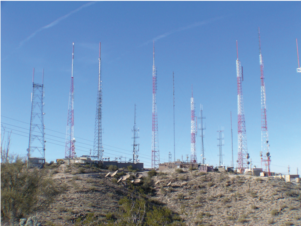
Figure 1. With this many emitters at a single site, measuring the contribution of each one would require cooperation from all organizations represented there, a highly unlikely event and the impetus for development of narrowband instruments.
